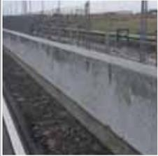
*PAS 68 rated predominantly surface mounted insitu concrete vehicle mitigation security solution. Can act as a foundation for lighting, CCTV masts and fences.*
