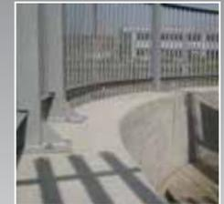
*By creating a curved corner detail embedded anchors can be avoided. Minimum radii are around 4.5m. Fences fixed to the top of radius barrier can also reflect a similar curve.*
