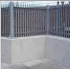
*Infinitely variable corner details can be provided to suit all required changes of barrier alignment. Fences affixed to the top can also reflect a similar arrangement.*
