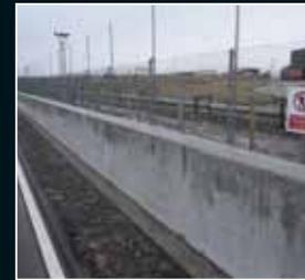
During the typical life cycle of the insitu concrete system the barrier is designed to provide a minimum 50-year maintenance free life; an extremely important consideration for many site operators where the disruption caused by routine maintenance or whole scale system replacement can be highly disruptive, compromise site security and of cause lead to increased operating costs.
